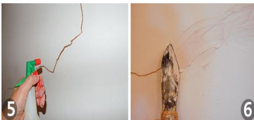
figure 4,2 joint filling
