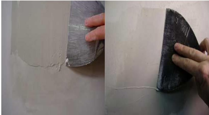
figure 5.6 apply second joint
