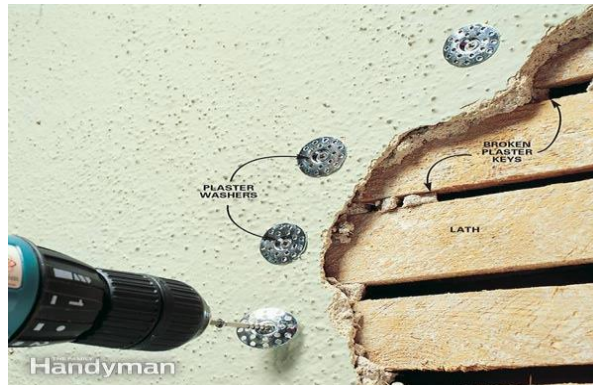
figure 1 repair sagging
