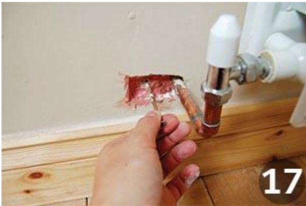
figure 4.4 cut off surface for hole
