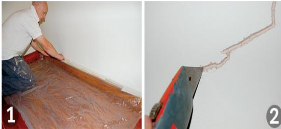
figure 4,1 repair crack
